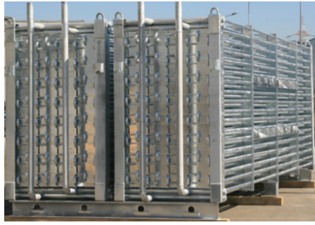
Figure 2.6: Chiller integrated TES for load shaving and shifting (Ragoowansi et al. 2023)
