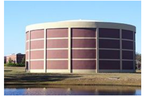
Figure 2.6: Chiller integrated TES for load shaving and shifting (Ragoowansi et al. 2023)
