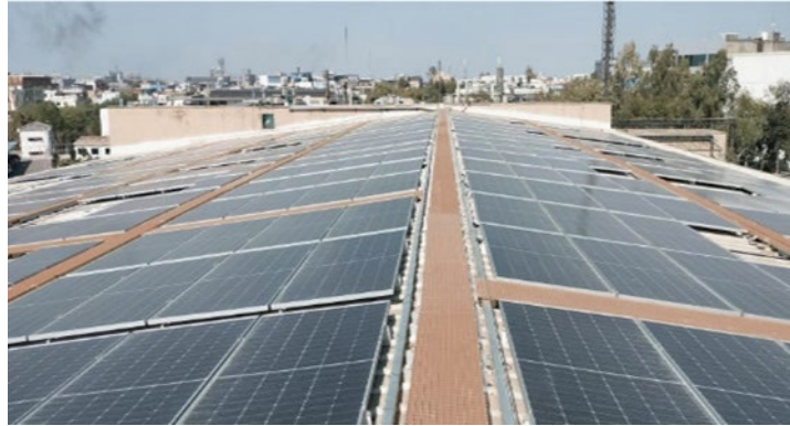
On Grid Roof mount Solar Photovoltaic Power Plant at Honeywell India factory
