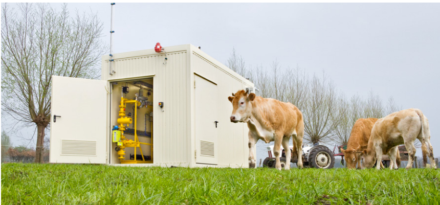
Figure 2.4: Biogas measurement, analysis and grid injection
